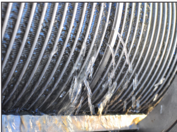
Low solids filtrate is removed from sludge fed to the SSD
