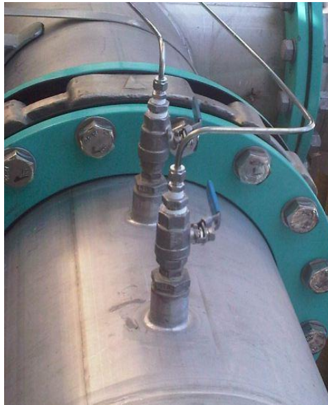
Figure 5 - Ball valve assembly
